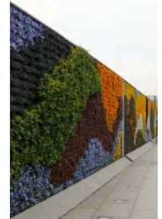
Green walls and facade treatments
